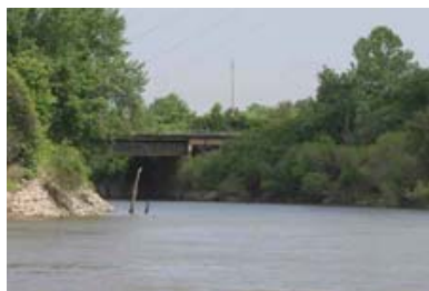
Confluence of the River Des Peres and Mississippi River: the concrete culvert becomes a real stream again, but what's in that water? MCE works to remediate urban watershed problems. Photo: Dale Dufer Studio
