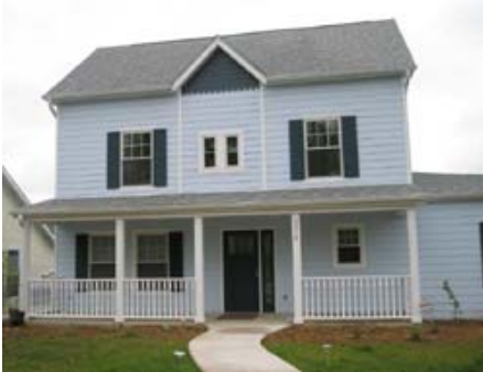
What does a high-performance certified-green home look? Like any handsome new home! Photo: Applied Energy Systems
