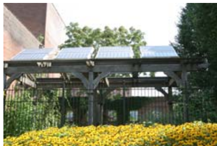
Solar panels power EarthWays Center's kitchen appliances and outdoor lighting. Photo: Dale Dufer
